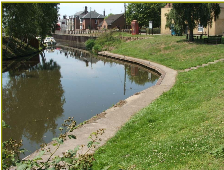
Photo 6: The boat basin, Outwell, Norfolk (application granted)
